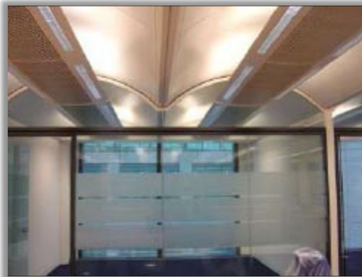
Figure 9 – Passive Multi-service Beams
