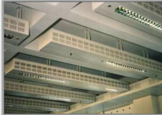
Figure 3 – Exposed Passive Chilled Beams
