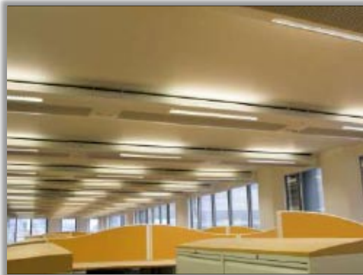
Figure 10 – Active Multi-service Beams
