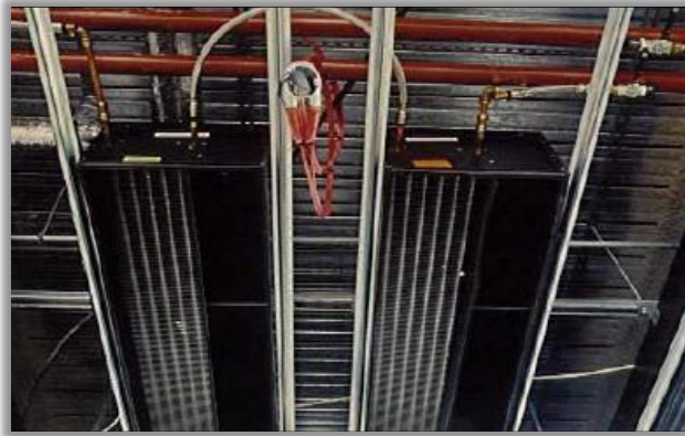
Figure 4 – Recessed Passive Chilled Beams
